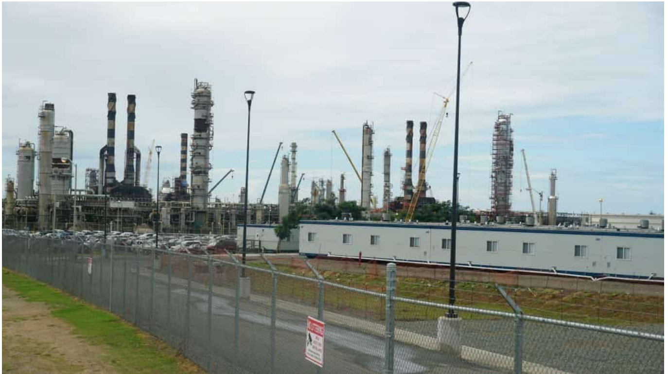
Man Camp near Limetree Bay By Ernice Gilbert, VIC
