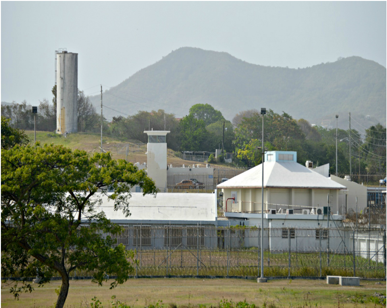
The John A. Bell Correctional Facility on St. Croix. By. V.I. CONSORTIUM
