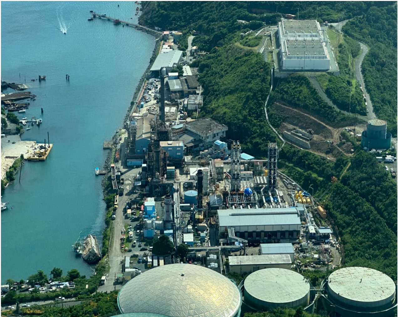
Aerial shot of the Randolph Harley Power Plant in St. Thomas, USVI. By. ERNICE GILBERT/ V.I. CONSORTIUM
