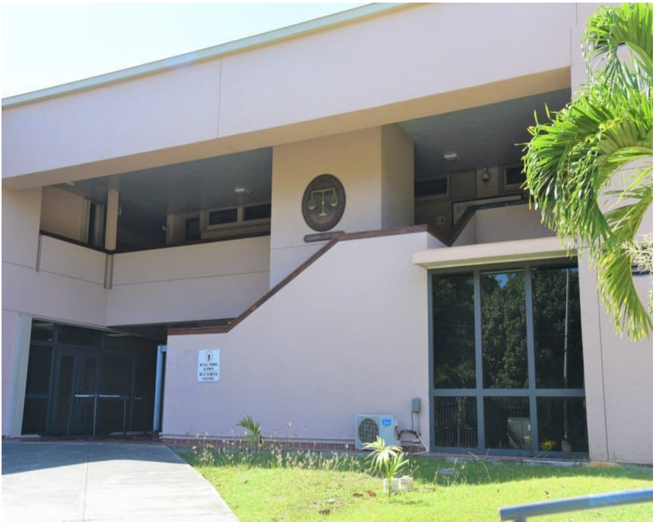
Superior Court building on St. Croix By. OFFICE OF DISASTER RECOVERY
