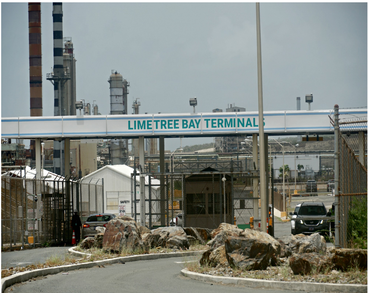
Limetree Bay Terminals By. Ernice Gilbert for VI Consortium
