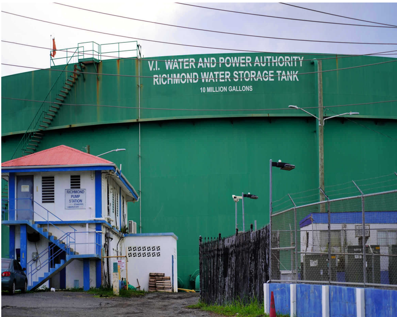
WAPA's Richmond Water Storage Tank. By. ERNICE GILBERT, V.I. CONSORTIUM.
