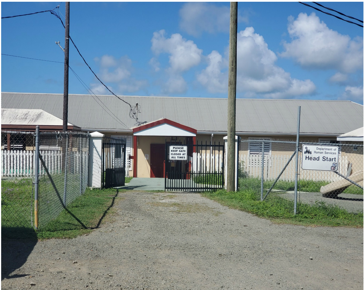
Head Start where incident took place (Ernice Gilbert, VIC)
