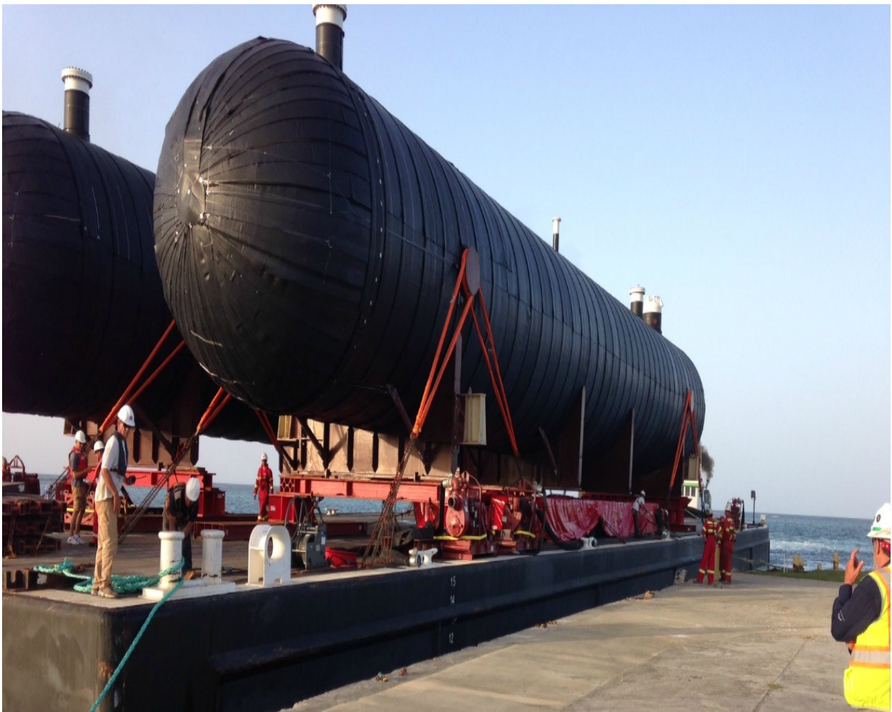
Propane tanks arrive at WAPA
