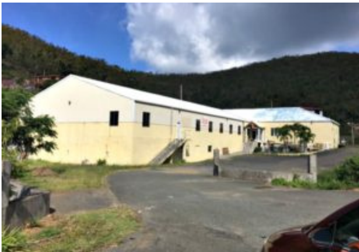
Office and Storage Space
