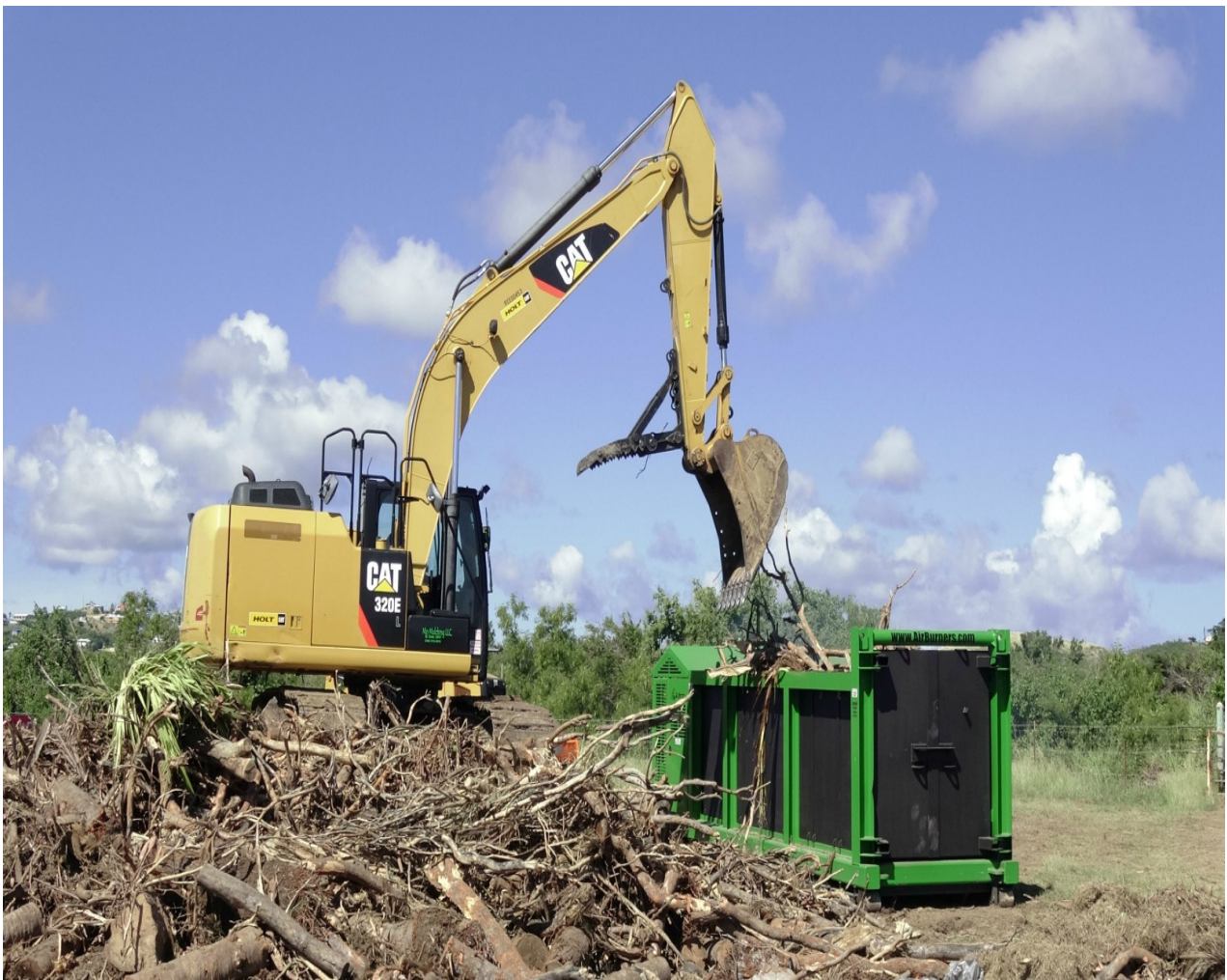
A CAT-branded excavator loads debris into an air curtain incinerator on the south shore of St. Croix on Dec. 13, 2017 (Ernice Gilbert, VIC)
