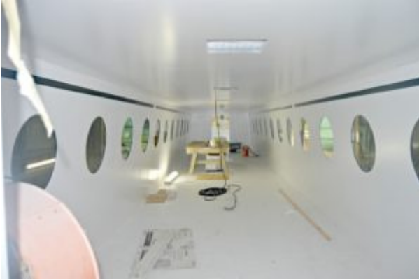
Inside the QE4, currently under construction
