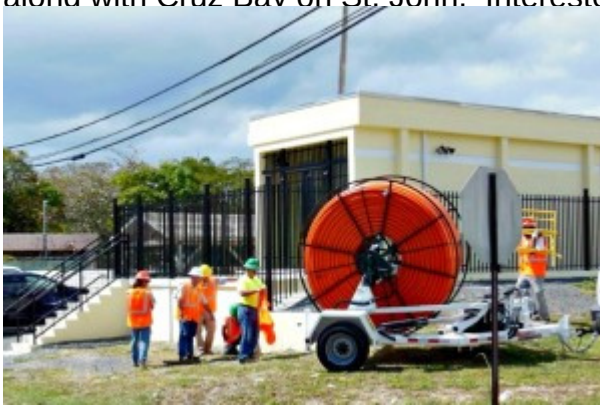
VINGN field employees work at a fiber access
