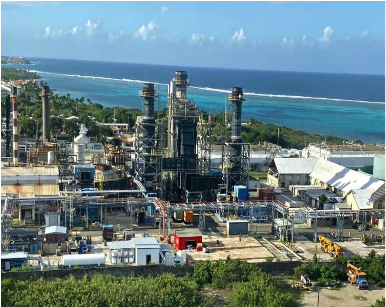
An aerial view of WAPA's powerplant in Richmond, St. Croix. By. ERNICE GILBERT, V.I. CONSORTIUM.
