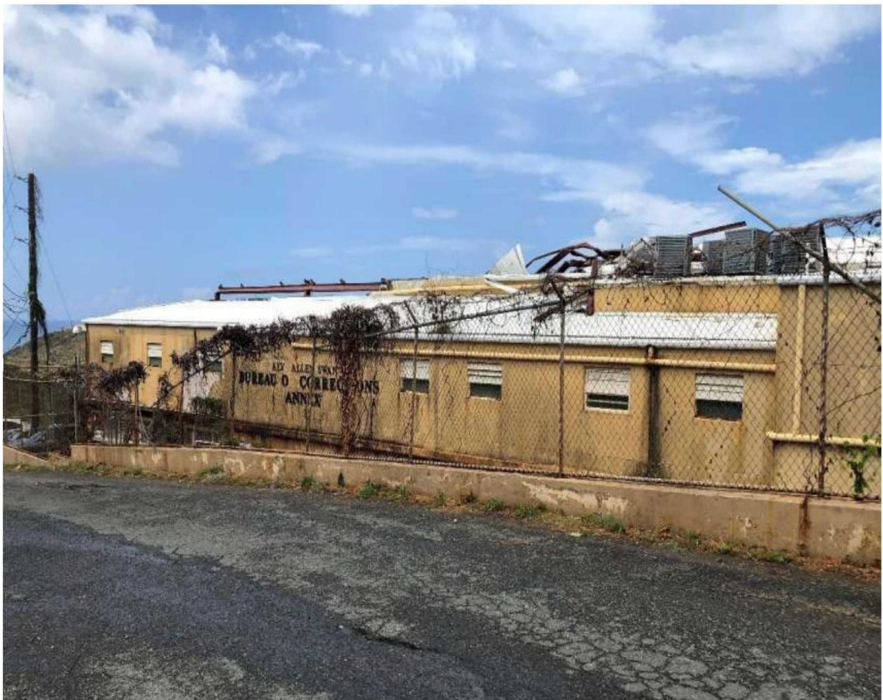
The condemned Alva A. Swan Correctional Annex in St. Thomas.
