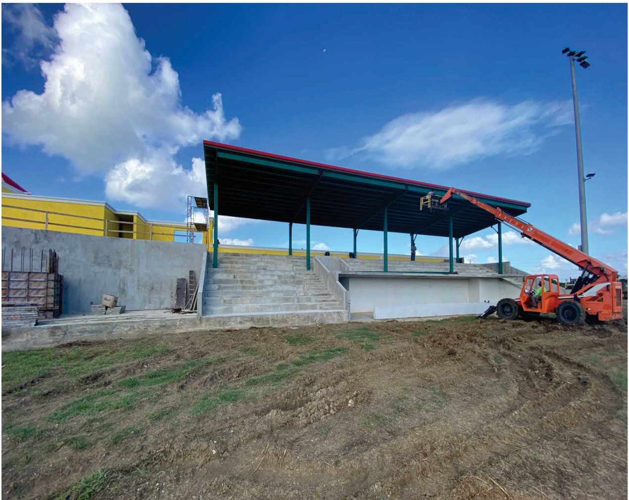
The left field bleacher roof of the Paul E. Joseph Stadium, currently under construction. By. DPW.
