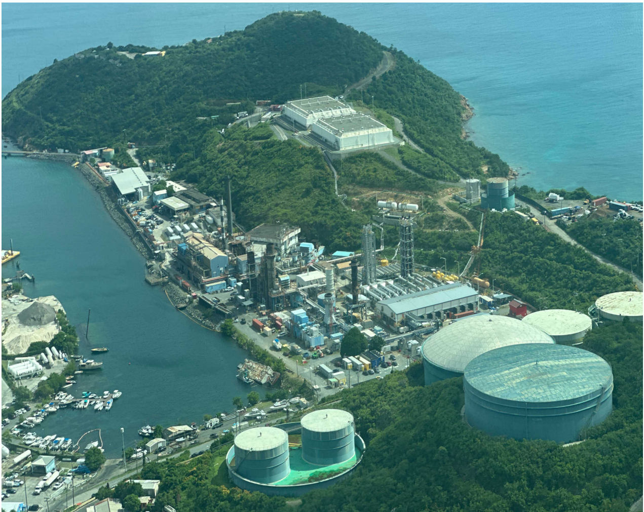
An aerial view of the Randolph Harley power plant in St. Thomas, USVI. By. ERNICE GILBERT, V.I. CONSORTIUM.
