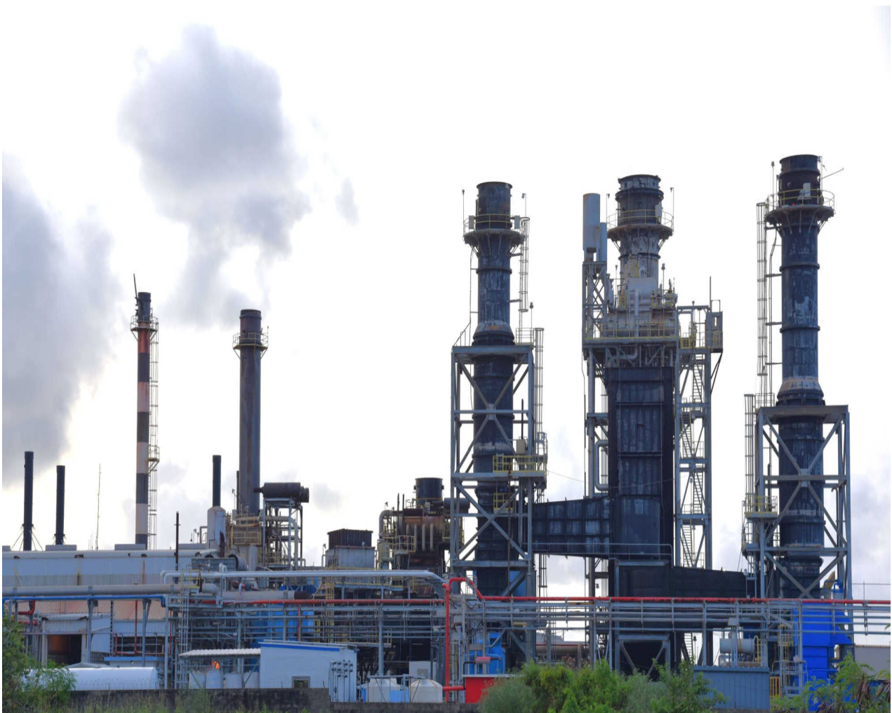
WAPA's Richmond power plant.
