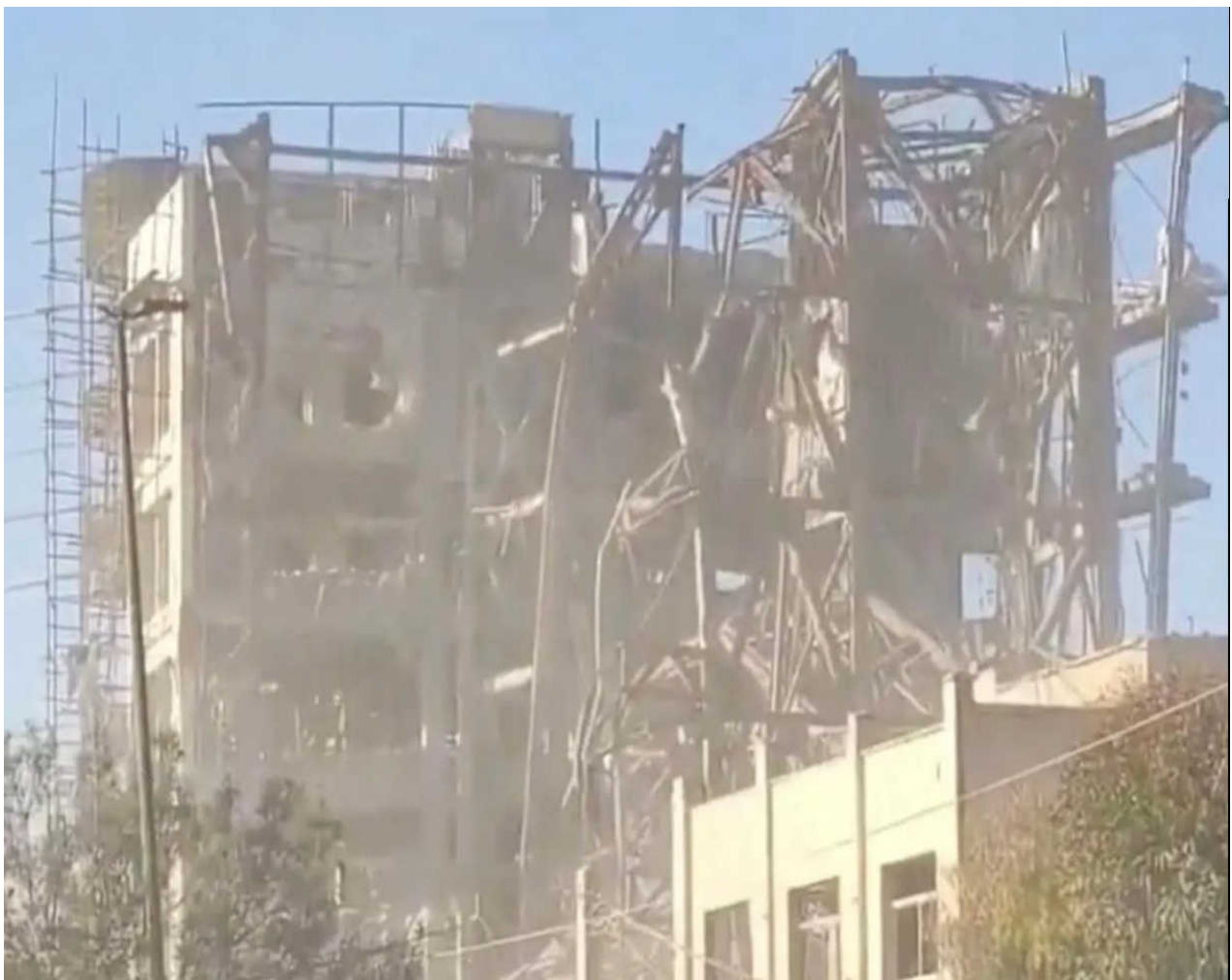
Damage to Iran's Assembly of Experts building in Qom from U.S.-Israel strikes.
