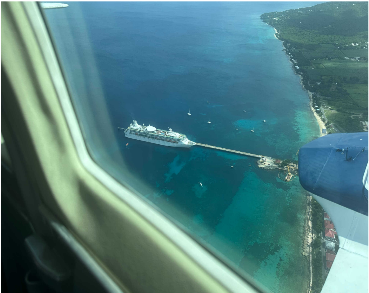
The Frederiksted Pier. By. V.I. CONSORTIUM.
