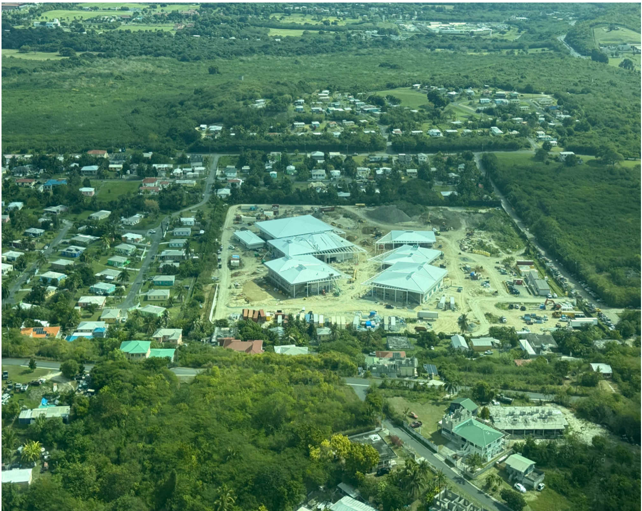
The Arthur A. Richards K-8 School under construction by MCN Build. By. V.I. CONSORTIUM.
