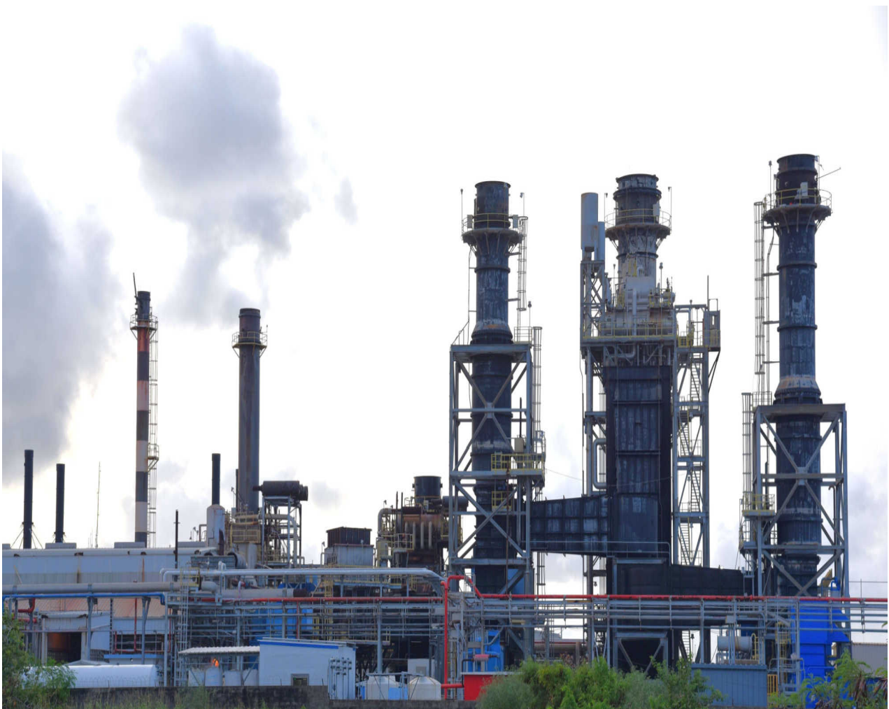
WAPA's Richmond power plant.
