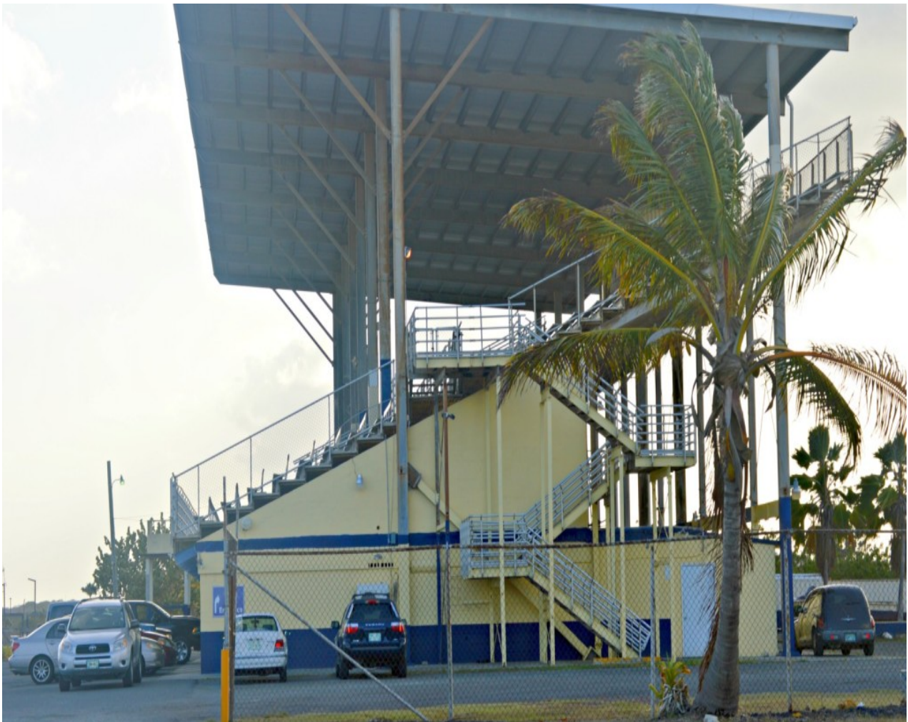
Randall “Doc” James Racetrack in June 2015 before it was demolished. By. ERNICE GILBERT, V.I. CONSORTIUM.
