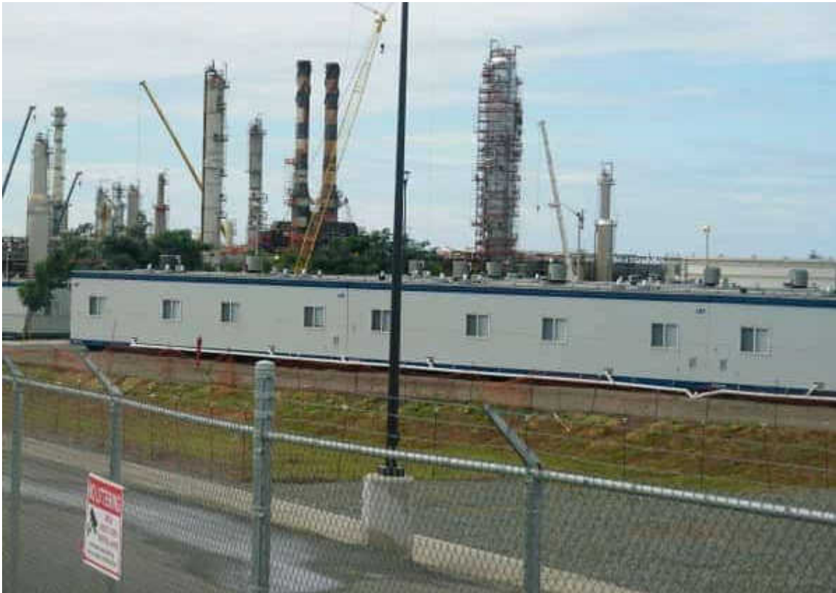
The PHRT Village, also known as the Man Camp, at the south shore refinery and terminal facility. (Credit: V.I. Consortium)
