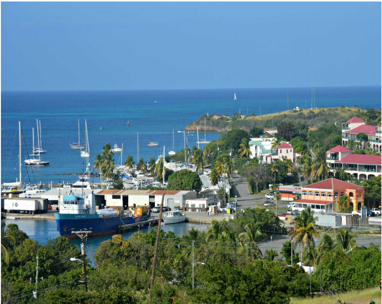
The Gallows Bay Marine Facility on St. Croix. By. V.I. CONSORTIUM.
