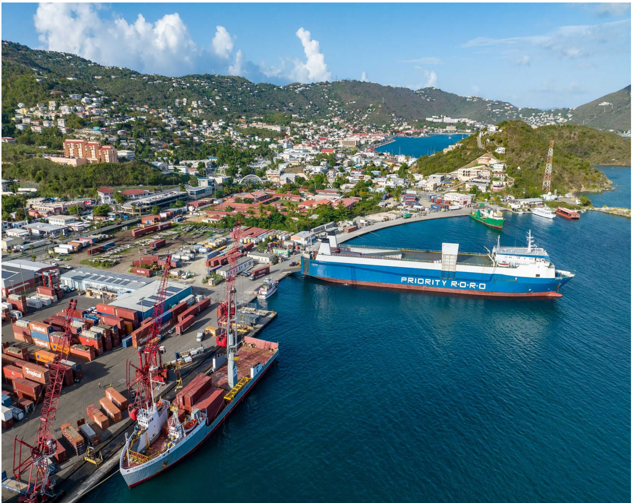
The Crown Bay Cargo Facility. By. TAFARI NELSON, VIPA ENGINEER.
