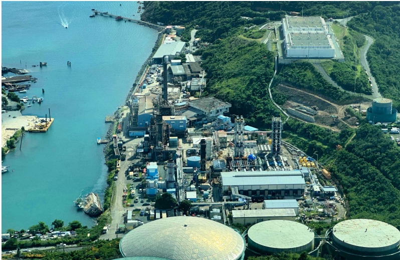
The Randolph Harley Power Plant in St. Thomas (Credit: Ernice Gilbert, V.I. Consortium)
