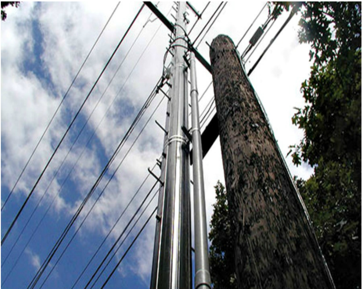
Composite pole installation in the U.S. Virgin Islands. By. FEMA
